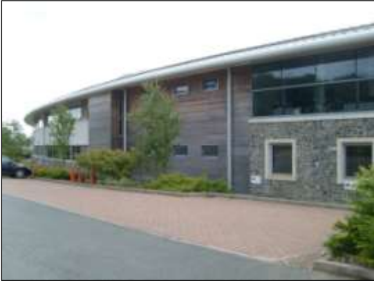
Figure 6 rear of Technium
